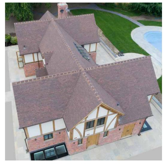
Canterbury handmade clay plain tiles in Loxleigh colour have been used to create an authentic roof for a new build historic-style cottage in the Denham conservation area. The self-build project, in the picturesque old English village, had to adhere to strict planning guidelines for roof height and use of materials due to the number of listed buildings along the same road.
